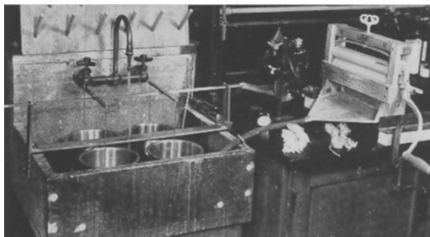
FIG. 2. Raw wool scouring train.
